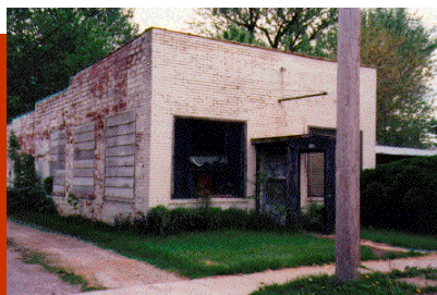
Old drycleaning facility
