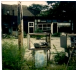
"Before" photo of 2759 West Washington
