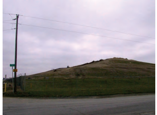
ERC/Coles County Landfill ceased accepting waste in April 2009, and a transfer station took its place at the same location, under a different owner/operator.
