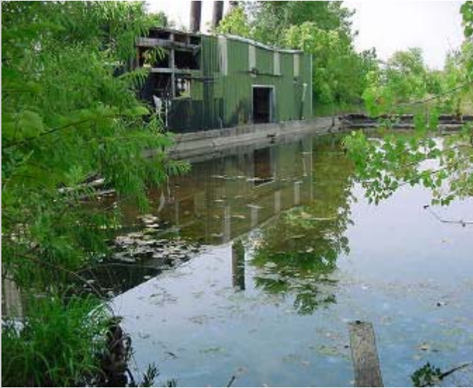
A railroad tie creosote treatment building and basin at the Jennison-Wright NPL site.
