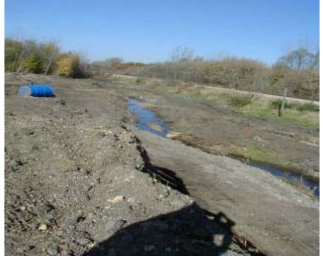
A drainage ditch at the Southeast Rockford Groundwater Contamination NPL Site.
