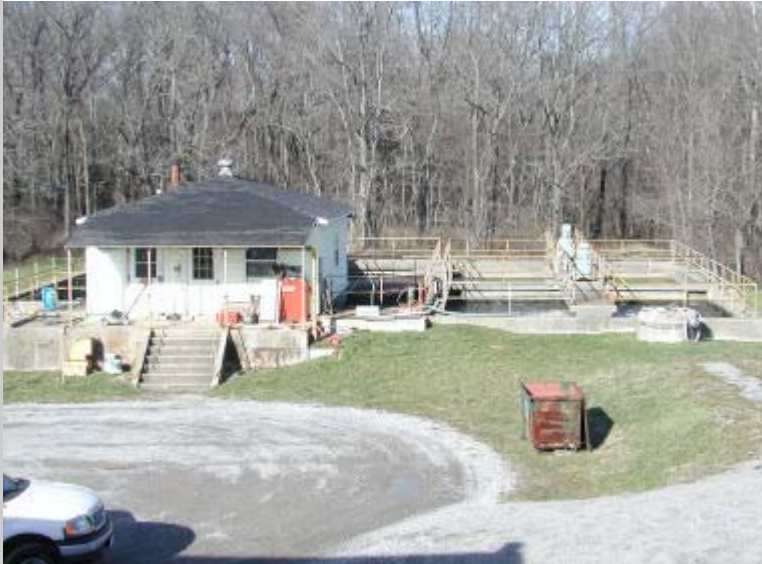
Crab Orchard National Wildlife Refuge NPL Site Waste Water Treatment Plant.
