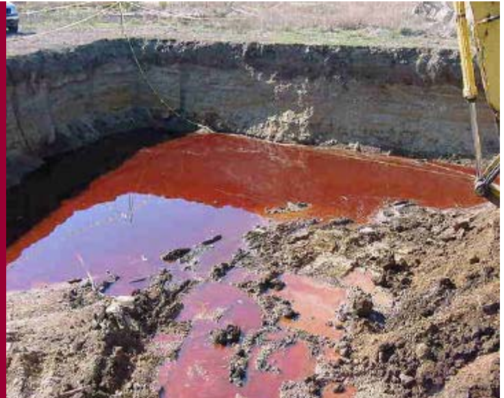
Trinitrotoluene (TNT)-contaminated groundwater (redwater) in an excavation at the Joliet Army Ammunition Plant NPL site.
