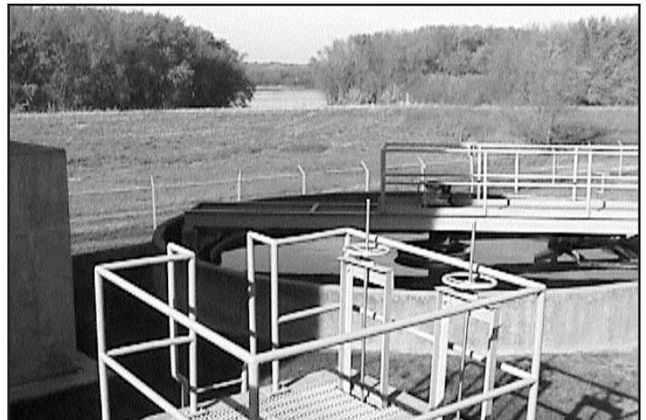
Fulton clarifier and receiving stream.
