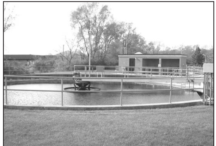
Secondary clarifier at the Weaton SD wastewater treatment facility.
