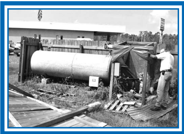
Assessing water supply hurricane damage in St. Tammany Parish, La.
